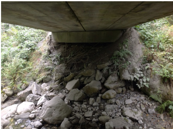
Right Bank Abutment when facing downstream
