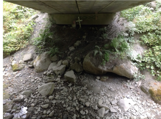
Left Bank Abutment when facing downstream
